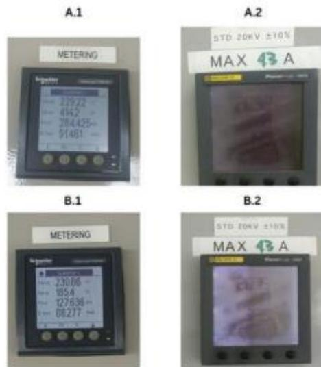
Gambar 4. Kondisi 1 PM Panel *Combiner* (A.1); Kondisi 1 PM Panel MVMDB (A.2); Kondisi 2 Panel *Combiner* (B.1); Kondisi 2 Panel MVMDB (B.2)
