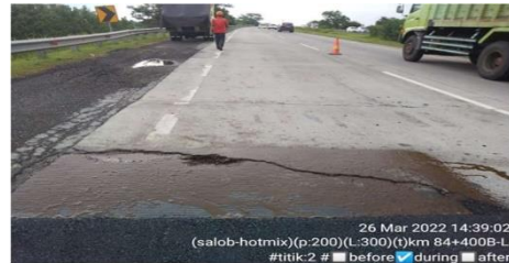
Gambar 5 Area Patching (ACBC)
