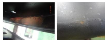
Gambar 4. 2. Jenis Defect Outflow : Karat
